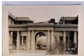
1458. California, Long Beach, Real Photo w/ DOPS P.C. back, Collapsed "Polytechnic High School" w/ Fallen Dome VF .. $25.00
