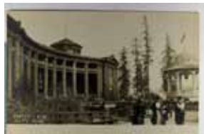
453. 1909 Alaska Yukon Pacific Expo., Real Photo, "Forestry Building" VF .. $15.00
