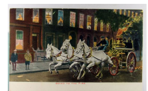
1585. Firefighting, "Going to the Fire" UB m cor wear Near VF ..$25.00
