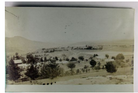
1549. South Africa, Used Capetown, Real Photo, Used 1908 m cor wear & m crs F-VF .. $25.00
