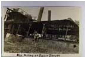
1537. Panama, Sunken Dredge, Real Photo w/AZO P.C. back wof & trimmed .. $20.00
