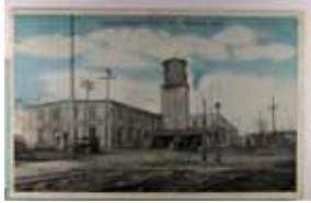
1202. Adv. Crow-Elkhart Motor Co., Indiana, Printed Photo WB cor wear & m face scrape Near F-VF .. $15.00
