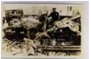
1391. California, Long Beach, 1933 Earthquake Aftermath, Real Photo, Non P.C. back m cor wear Near VF .. $15.00
