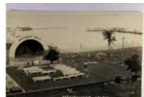
1480. Michigan, Menominee, Real Photo w/ EKC P.C. Back m cor wear Near VF .. $20.00
