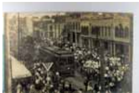
1432. Street-Car, Owner ID as Inaugural Run of TMER&L Co. into Watertown, Wisconsin, Real Photo, Used 1908 VF .. $80.00
