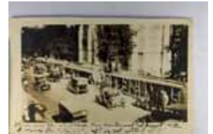
1010. Labor Related, "Streetcars Overturned and Burnt During The Strike", Real Photo w/AZO P.C. back flts .. $80.00
