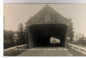
1434. Maine, The Forks, Real Photo w/ Covered Bridge VF .. $15.00
