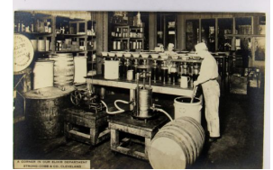
10. Adv. Strong-Cobb & Co. Medicine Factory, Real Photo w/ AZO P.C. back, Interior View w/ Machinery, Cleveland, Ohio VF .. $100.00
