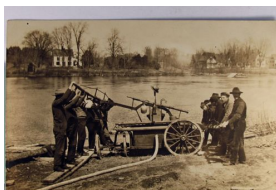
276. Water Pumping Equipment, Real Photo w/ AZO P.C. back, Owner ID as Weymouth, Massachusetts VF .. $95.00
