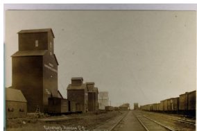
1492. South Dakota, Hudson, Real Photo w/ AZO P.C. back, "Elevators" VF .. $25.00
