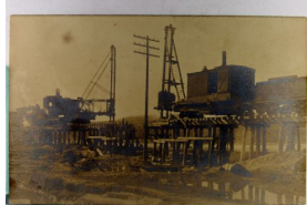
1348. Railroad Bridge Construction, Real Photo VF .. $20.00
