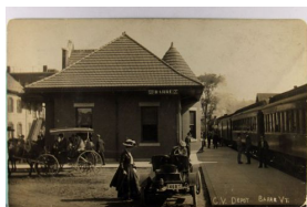
1358. Depot, Barre, Vermont, Real Photo, Used 1911 crs & wear F .. $30.00
