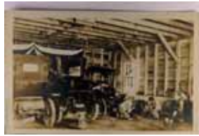
1248. Nassau Garage Interior, Real Photo w/ AZO P.C. back, Nassau, New York VF .. $100.00
