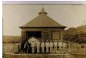
1479. Oregon, Newport, Real Photo, Life-Saving Station, Used Same 1913 edge flt F .. $15.00
