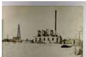
294. Construction Scene, Real Photo w/ AZO P.C. back F-VF .. $15.00
