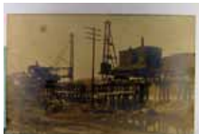
1348. Railroad Bridge Construction, Real Photo VF .. $20.00
