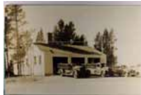
1509. Wisconsin, Camp McCoy, Real Photo w/ EKC P.C. back, Fire Station VF .. $15.00
