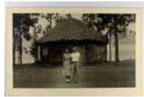
1569. Congo, Ibinja Island, Real Photo, w/ Message from Missionaries, Used Bukavu 1955 m cor wear F-VF .. $20.00
