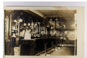
264. Bar Interior, Real Photo w/ Velox P.C. back, Owner ID as Michigan edge st Near VF .. $20.00
