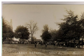
1412. Ohio, Leroy, Real Photo w/AZO P.C. back, "Leroy School" m cor cr Near VF .. $35.00
