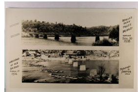
1419. Pennsylvania, Apollo Bridge Collapse, Real Photo w/ EKKP P.C. back, Dated 1938 VF .. $20.00
