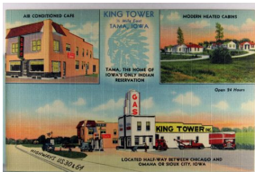
1176. Adv. King Tower Gas Station, Etc., Sioux City, Iowa, Curt Teich Pub. L VF .. $10.00
