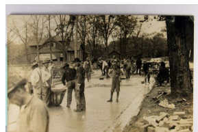
272. Road Construction, Real Photo, Used Ottawa, Illinois, 1914 m cor cr VF .. $15.00
