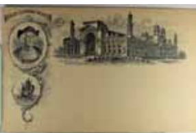
406. 1893 Columbian Expo., Koehler Pub. Official Ser. on Gov't Postals, Electrical Bld. VF .. $50.00
