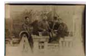
270. Workmen w/ Machinery, Real Photo w/ Cyko P.C. back m cor wear F-VF .. $40.00
