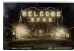
1389. Montana, Great Falls, Elks Convention, Real Photo, Used 1908, "Central Ave by Electric Light" m cor wear Near VF .. $25.00
