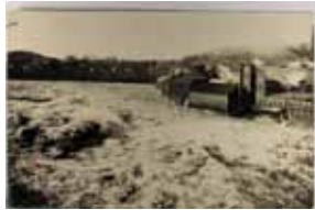
1432. Vermont, Bellows Falls, Real Photo, Used, Flood Scene VF .. $15.00
