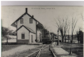
1426. Depot, Warner, New Hampshire, Printed Photo DB VF .. $15.00
