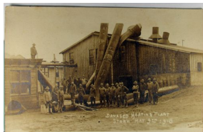
283. Disaster Real Photo w/ Kruxo P.C. back, "Damaged Heating Plant" Dated May 9th, 1918 m cor cr VF .. $25.00
