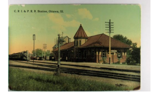
1415. Depot, Ottawa, Illinois, Tinted Printed Photo DB wear Near F-VF .. $10.00
