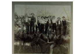
311. Men Working w/ Thatch, Real Photo on Board, Non P.C. m cor crs & m edge cr F-VF .. $20.00
