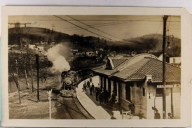
1411. Depot, Owner ID as Near Grafton, West Virginia, Real Photo, Used 1918 cor flt F .. $30.00
