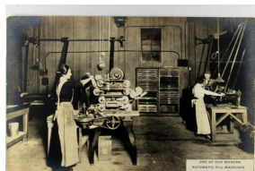
8. Adv. Strong-Cobb & Co. Medicine Factory, Real Photo w/ Non P.C. back, Interior View w/ Machinery, Cleveland, Ohio VF .. $75.00
