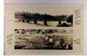
1520. Pennsylvania, Apollo Bridge Collapse, Real Photo w/ EKKP P.C. back, Dated 1938 VF .. $25.00
