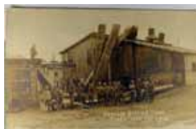
283. Disaster Real Photo w/ Kruxo P.C. back, "Damaged Heating Plant" Dated May 9th, 1918 m cor cr VF .. $25.00
