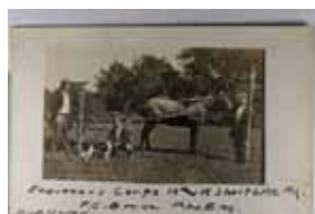
1389. A&A Shortline Ry, Engineer Corp., Real Photo w/ AZO P.C. back, incl. Surveying Equipment, Dated 1911 Near VF .. $125.00
