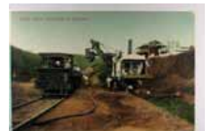
1565. Panama, Gorgona, "Steam Shovel", Tinted Photogravure, Used Same VF .. $10.00
