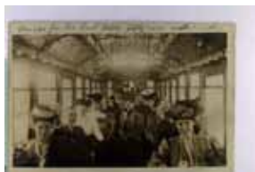
1392. Train Car Interior, Real Photo DB w wof & m edge wear F-VF .. $30.00
