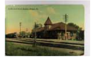
1415. Depot, Ottawa, Illinois, Tinted Printed Photo DB wear Near F-VF .. $10.00
