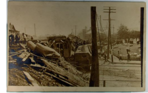
1425. Train Wreck, Real Photo, Owner ID as Bridgeport, Connecticut, used Same 1911 m cor wear Near VF .. $50.00
