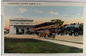
1422. Lackawanna Station, Elmira, New York, Tinted Printed Photo WB VF .. $20.00
