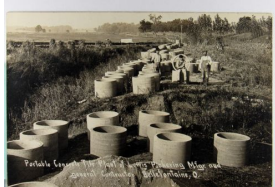
1516. Ohio, Bellefontaine, Real Photo, "Concrete Plant" VF .. $25.00
