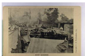
993. 1932 Bonus Army, Washington DC, "Roof Gardens", Printed Photo m cor wear Near VF .. $40.00
