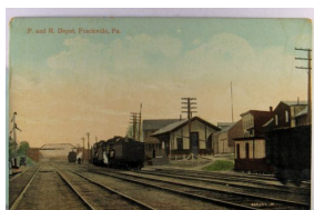
1428. Depot, Frackville, Pennsylvania, Tinted Printed Photo, Used 1914 DB cor wear Near F-VF .. $15.00
