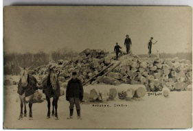
1501. Michigan, Pellston Studio, Real Photo, Lumber Related m cor wear F-VF .. $20.00
