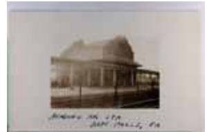
1420. Depot, East Falls, Pennsylvania, Real Photo w/ AZO P.C. back m wof VF .. $60.00
