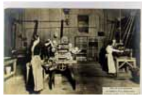
6. Adv. Strong-Cobb & Co. Medicine Factory, Real Photo w/ Non P.C. back, Interior View w/ Machinery, Cleveland, Ohio VF .. $75.00
