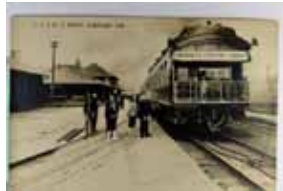
1408. Train Depot, Elkhart, Indiana, Real Photo Near VF .. $75.00
