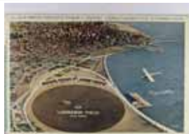
1371. Airport, Lindbergh Field, San Diego, California, Used 1930 WB m cor wear F-VF .. $15.00
