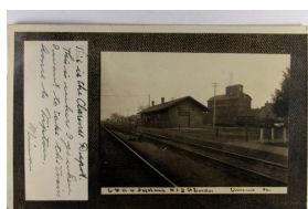
1368. Train Depot, Clarkville, Pennsylvania, Real Photo w/ Karbo P.C. back, used 1909 wof F-VF .. $90.00
