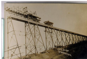
1351. Railroad Bridge Under Construction, Real Photo w/ Kruxo P.C. back, "Lethbridge Alta" VF .. $25.00
