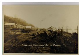
1448. Iowa, Keokuk, Dam Construction, Real Photo w/ Artura P.C. back VF .. $20.00
