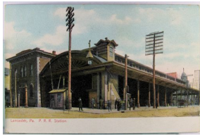
1381. Depot, Lancaster, Pennsylvania, Tinted Photogravure UB m cor wear VF .. $15.00
