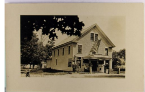
1505. New Hampshire, Effingham Falls, Ice Cream Parlor, Real Photo w/ Defender P.C. back VF .. $25.00
