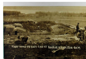
1449. Iowa, Keokuk, Dam Construction, Real Photo w/ AZO P.C. back m cor wear VF .. $20.00
