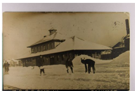
1356. Depot, Calumet, Michigan, Real Photo, used 1910 cor wear & m cof Near F-VF .. $40.00
