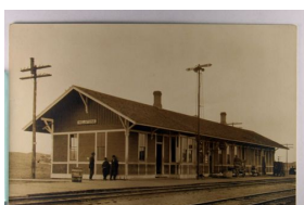
1366. Depot, "Melstone", Montana?, Real Photo w/ AZO P.C. back m cor wear Near VF .. $100.00
