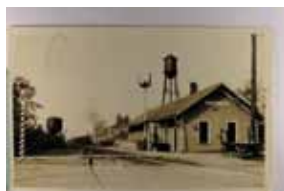
1363. Depot, Marion, Michigan, Real Photo, Used Same 1947 m edge tear & cor wear F .. $25.00
