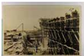
1447. Iowa, Keokuk, Dam Construction, "Mississippi River Power Co." Real Photo w/ Artura P.C. back m wof VF .. $20.00
