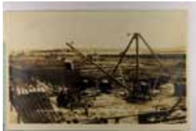
1451. Iowa, Keokuk, Dam Construction, Real Photo w/ Kruxo P.C. back m cor wear Near VF .. $20.00
