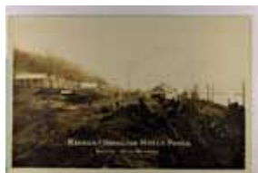
1448. Iowa, Keokuk, Dam Construction, Real Photo w/ Artura P.C. back VF .. $20.00
